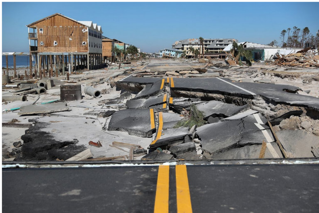
State Road 98, torn up after Hurricane Michael, in Mexico Beach, FL, Oct. 12. PHOTO: JOE RAEDLE/GETTY IMAGES
