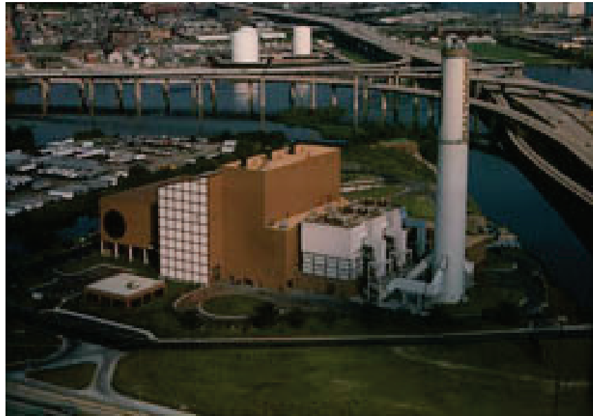
Baltimore RESCO (Refuse Energy Systems Company) Plant Russell Street & U.S Interstate 95 (shadow of Ravens Stadium)
