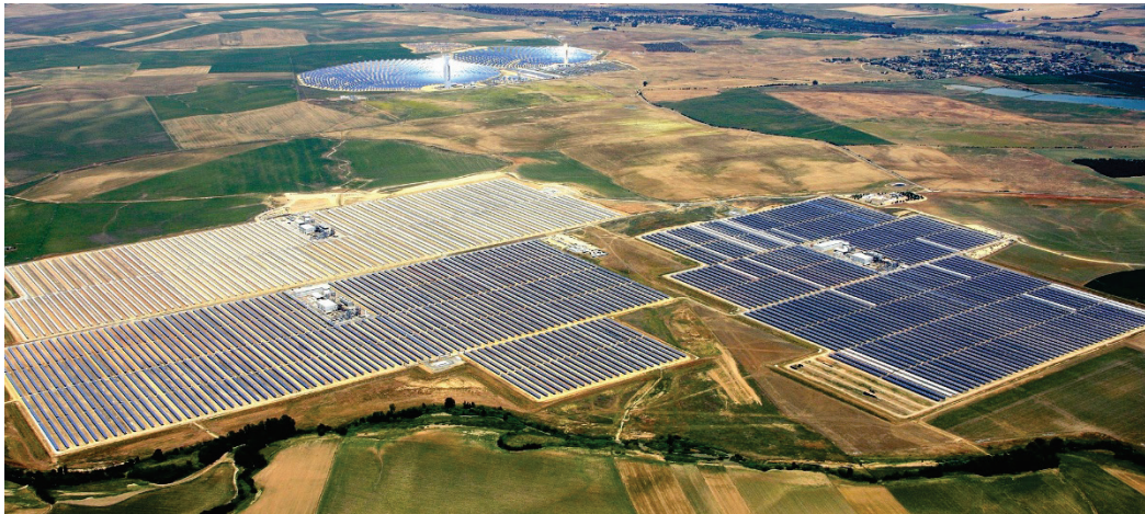
Left: Parabolic troughs (150 MW total) and two towers (30 MW) of the first three units of Solnova power station, Southern Spain.
