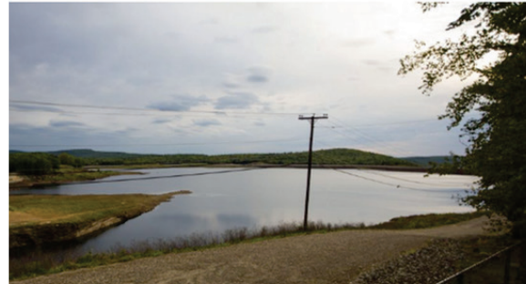
The upper reservoir is the battery that powers the Northfield Mountain pumped hydroelectric station. (Jesse Costa/WBUR)
